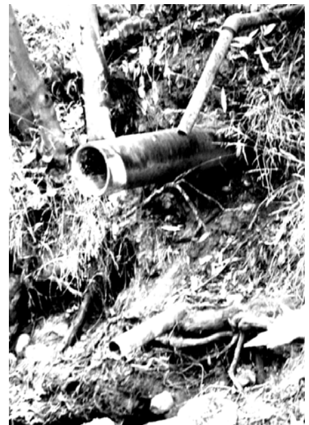
Outfalls on Strawberry Creek near Sather Gate, UC Berkeley.
